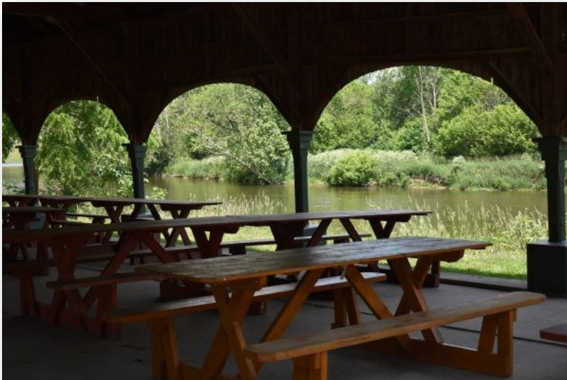
The arches of the Lower Spencer Shelter (as pictured above) are a significant architectural feature of this shelter.
