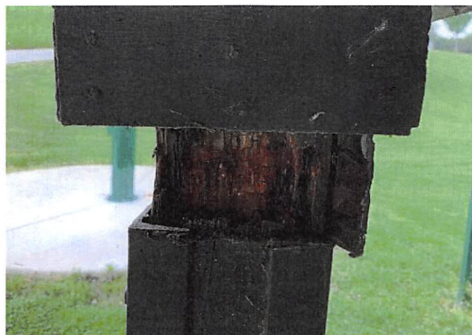
Figure 10: Rotten Post
