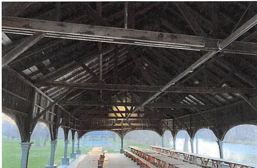
Figure 4: Overall Roof Structure
